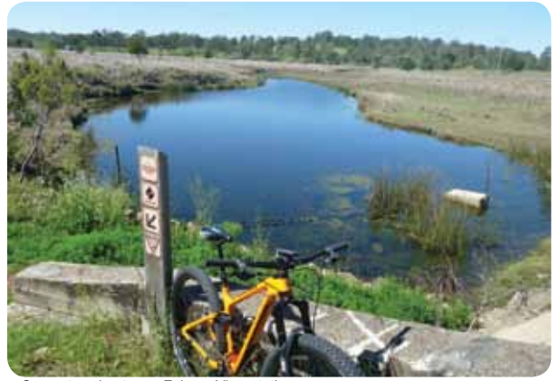
Concrete culvert near Fairney View station
