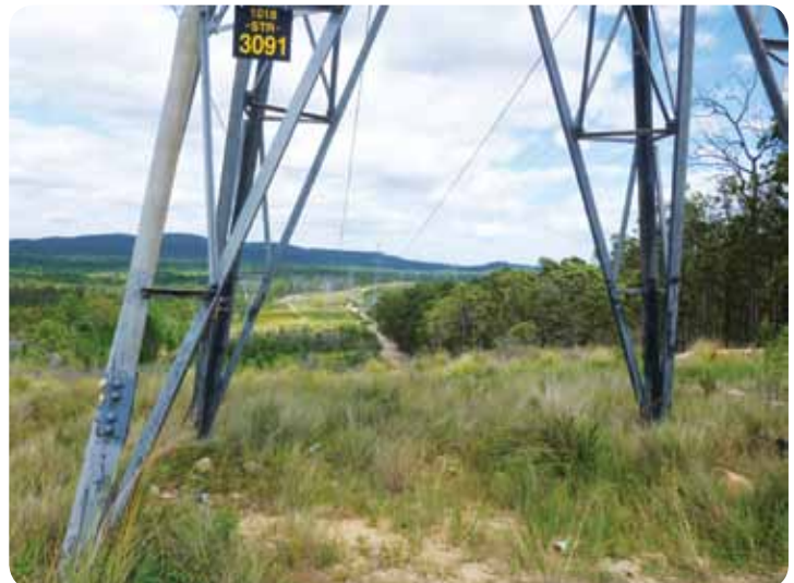
View to the west overlooking Yarrabilba from the power pylons
